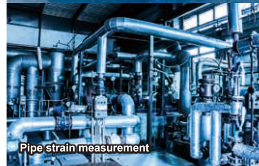
Brake and pipe strain measurement
